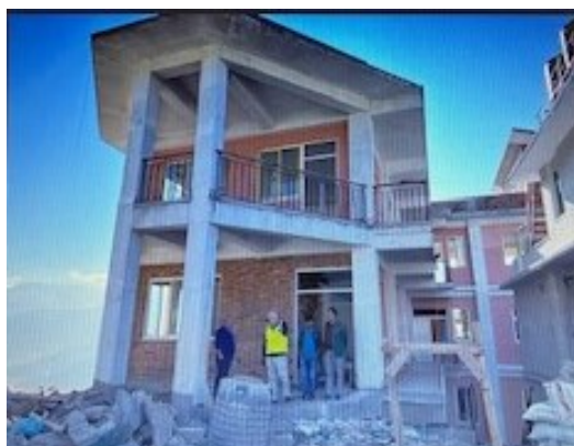
Hospital building in progress
